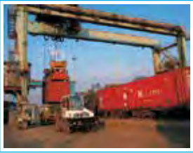
Top-notch Logistics & Service Facilities
