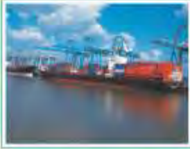
Deepened & Widened Channel
