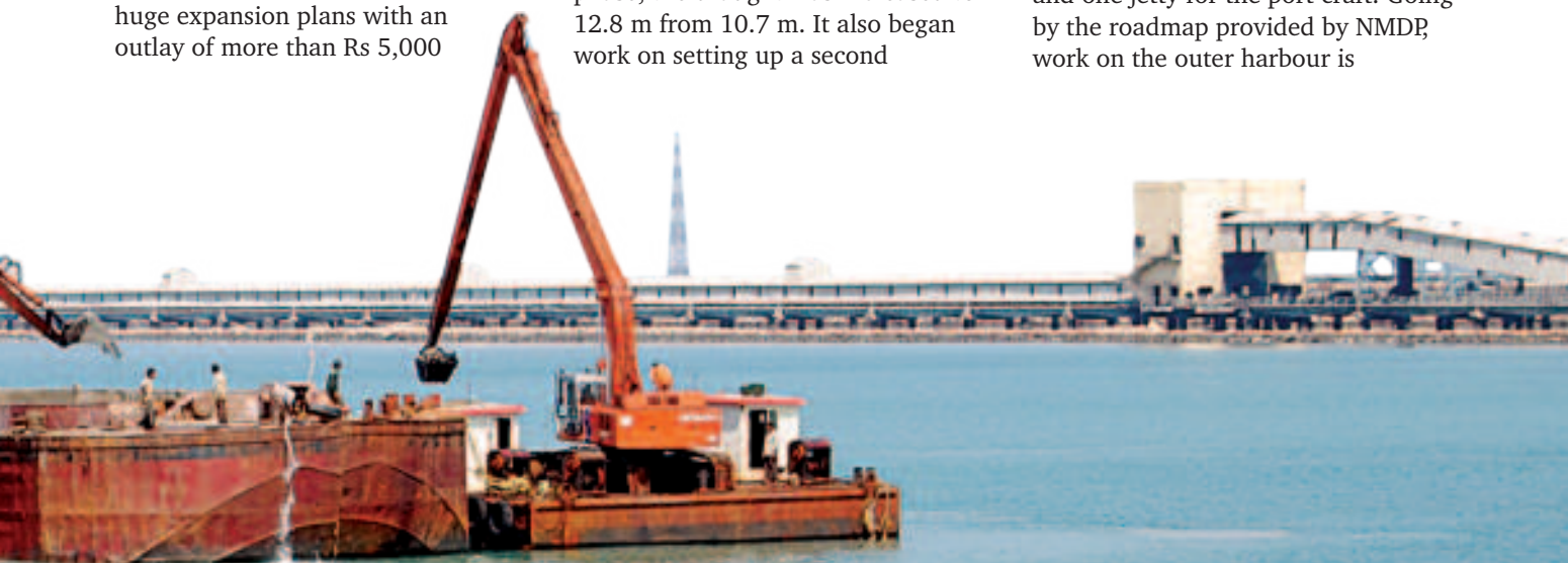
Dredging in full swing: Tuticorin Port has taken up dredging in the entry channel and alongside berths as part of its ambitious expansion plan.
