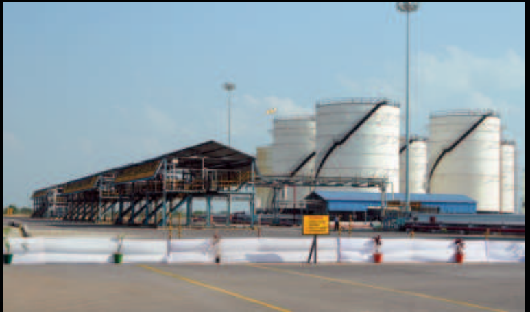
The marine liquid terminal at Ennore Port.
