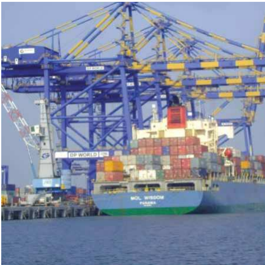
ICTT IS DESIGNED FOR A DRAFT OF 14.5 METRES FOR HANDLING CONTAINER SHIPS OF 8000+ TEU CAPACITIES
