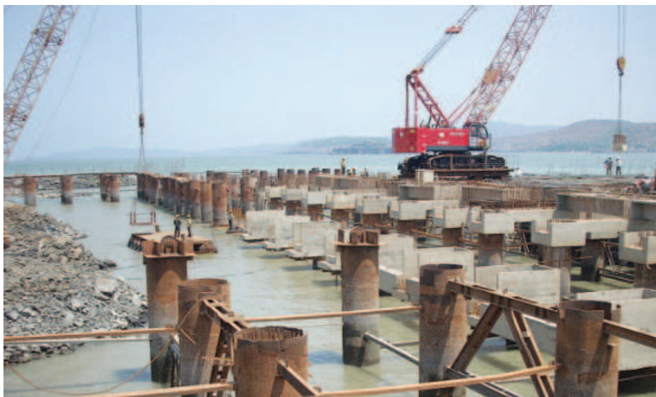
Construction of berths in progress
