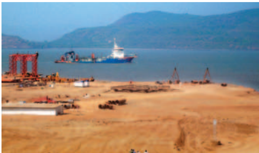
Sprucing up: Construction work being carried out at Dighi Port.
