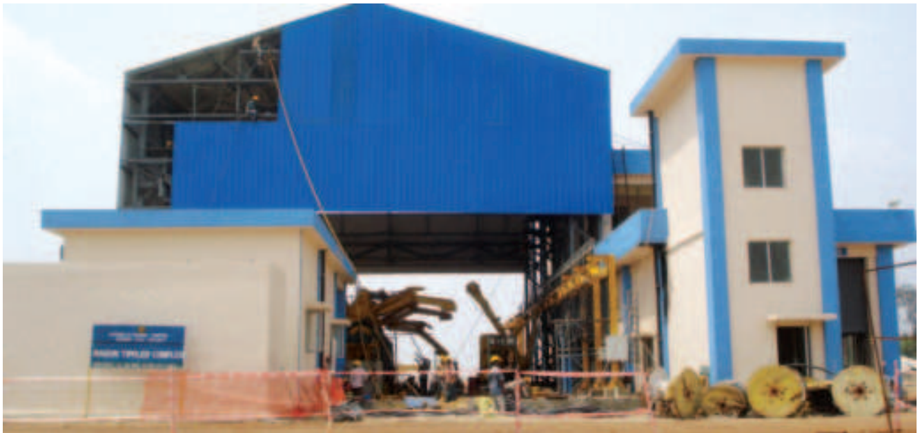
The wagon tippler complex in the port vicinity.
