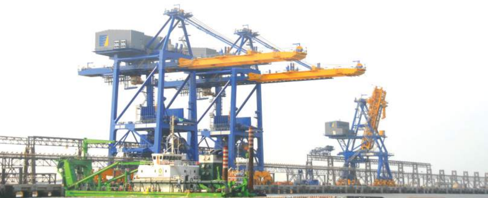
Coal unloading and iron ore loading equipment at the upcoming Dhamra Port in Orissa.
