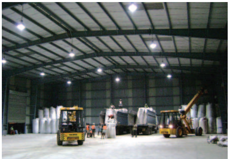
Karaikal Port aims to have 620,000 square metre of covered and uncovered storage space within the premises.
