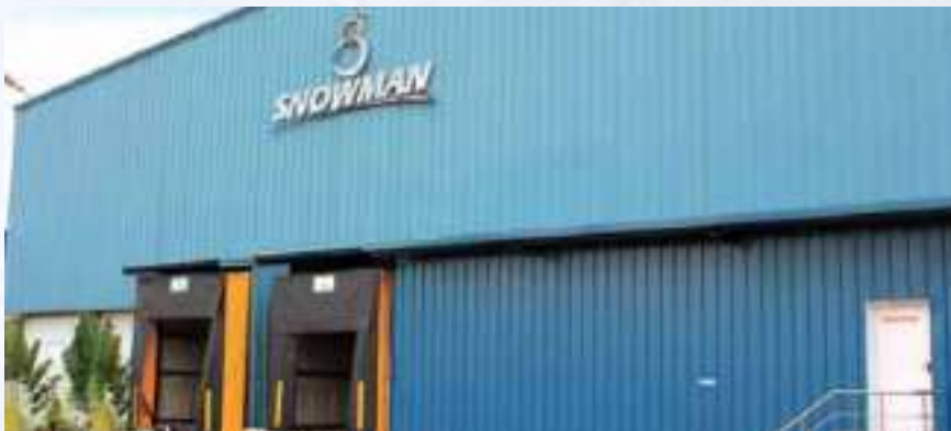
ALL SNOWMAN WAREHOUSES HAVE BEEN BUILT USING G+4 RACKING SYSTEMS
