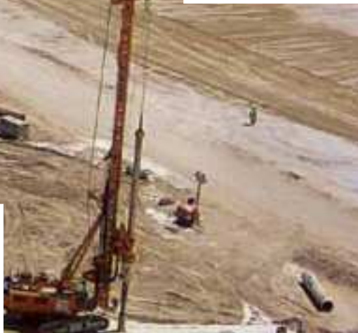
Piling work - Qatar
