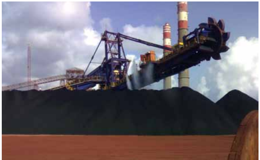
CARGO HANDLING FACILITIES AT THE PORT ARE A DELIGHT TO CUSTOMERS
