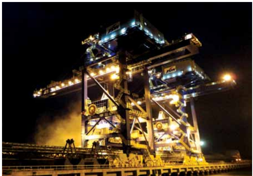
AFTER THE EXPANSION, 10 BERTHS WILL HANDLE 50 MT OF CARGO
