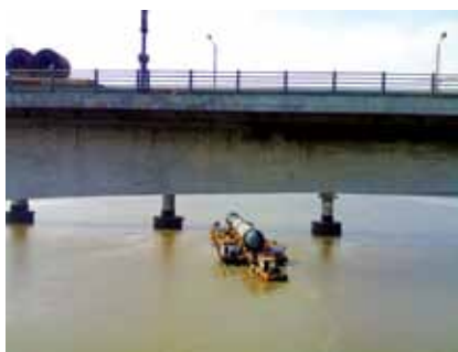
250-MT SINGLE CARGO BEING TRANSPORTED BY BARGE VIA VASHI BRIDGE TO MUMBAI PORT. THIS IS NOT POSSIBLE TO TRANSPORT BY ROAD DUE TO WEIGHT AND SIZE
