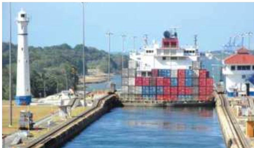
AFTER THE PANAMA CANAL OPENS, IT IS PROJECTED THAT THE NUMBER OF CONTAINERSHIPS AND BULK CARRIER TRANSITS WILL ACTUALLY FALL AS LARGER SHIPS DISPLACE SMALLER ONES.
