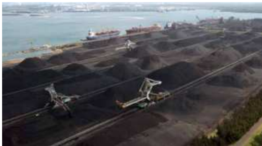
THE RICHARDS BAY COAL TERMINAL (RBCT), LOCATED IN THE RICHARDS BAY HARBOUR ON THE INDIAN OCEAN COAST OF SOUTH AFRICA, IS THE LARGEST COAL EXPORT FACILITY IN AFRICA. SOUTH AFRICA'S ECONOMICALLY RECOVERABLE COAL RESERVES ARE ESTIMATED AT 55 BILLION TONNES.
