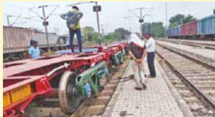
Driving Logistics with 18,000 + Wagons on track at 190 Locations
