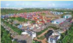
67 terminals Including 16 MMLPs setup across the country
