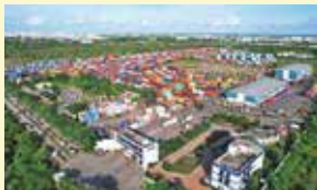
67 terminals Including 16 MMLPs setup across the country
